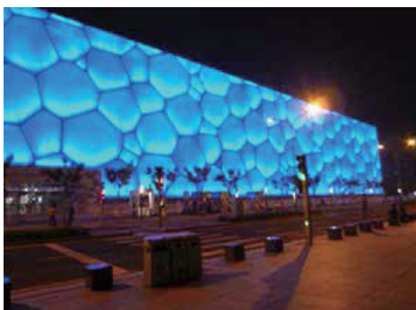
Beijing National Aquatics Center (Water cube)
